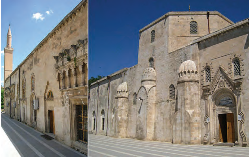
Figure 9.3 Two views of the exterior of the Friday Mosque of Mayyāfāriqīn.
